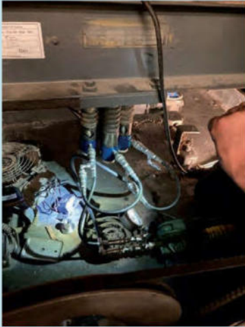
Figure 12: A hydraulic rope tension equalizer in use
